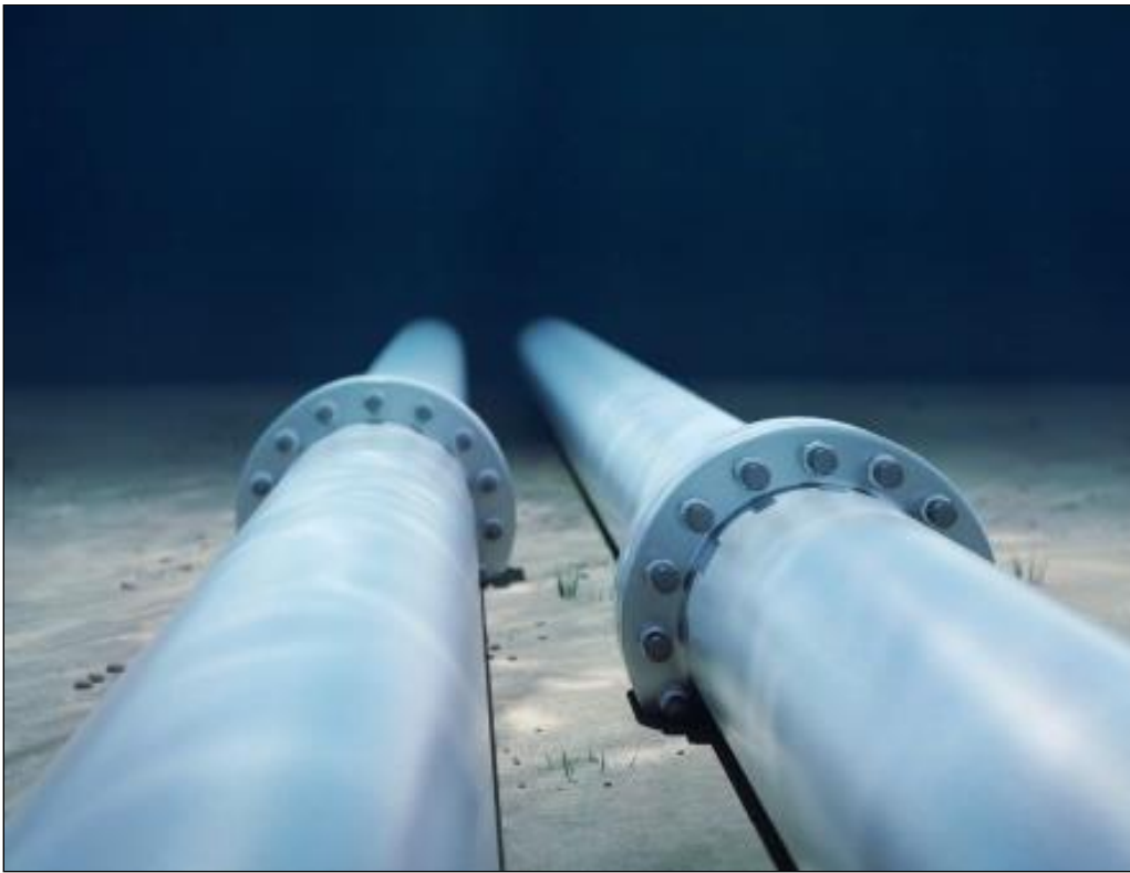
View of an underwater pipeline.
