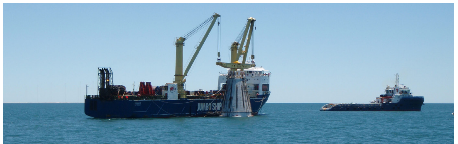
Image 1. Installation of the DTM in 2008
