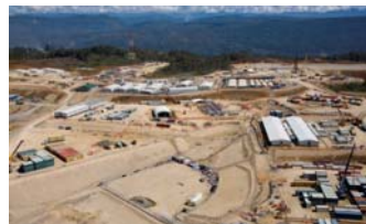
Hides gas conditioning plant
