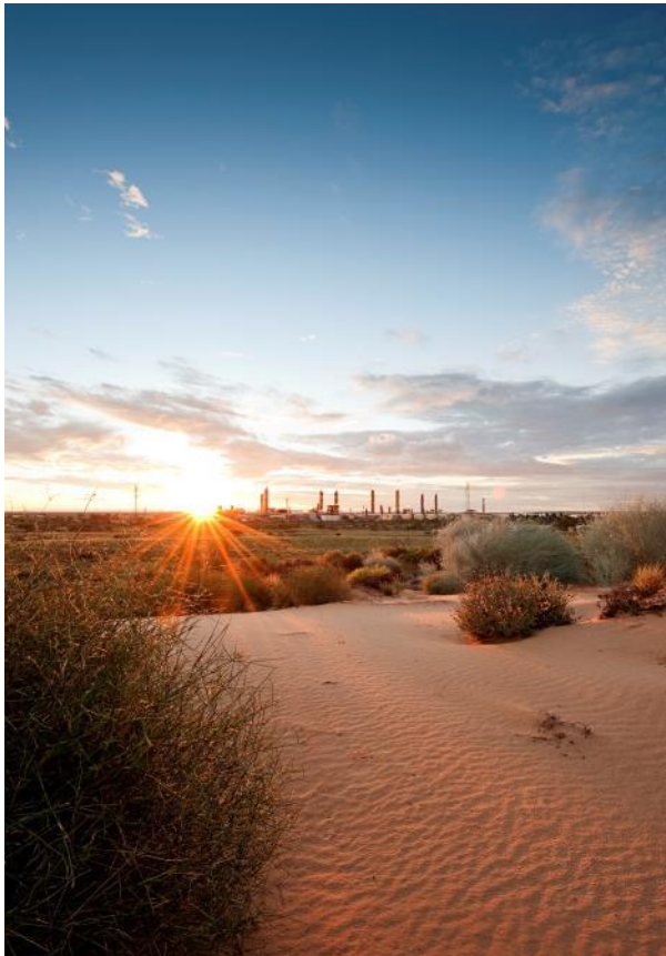
Moomba Plant, Cooper Basin
