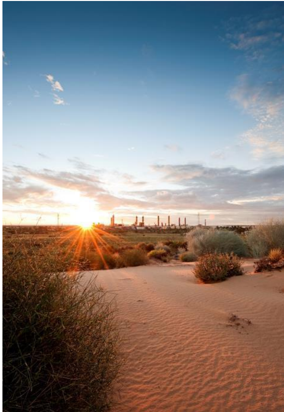
Moomba Plant, Cooper Basin
